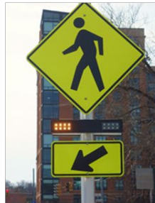
b: Rectangular Rapid Flashing Beacon (RRFB)
